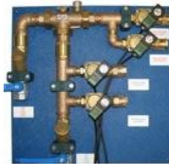
Control boards for each basin in housing with pressure switches mounted.
